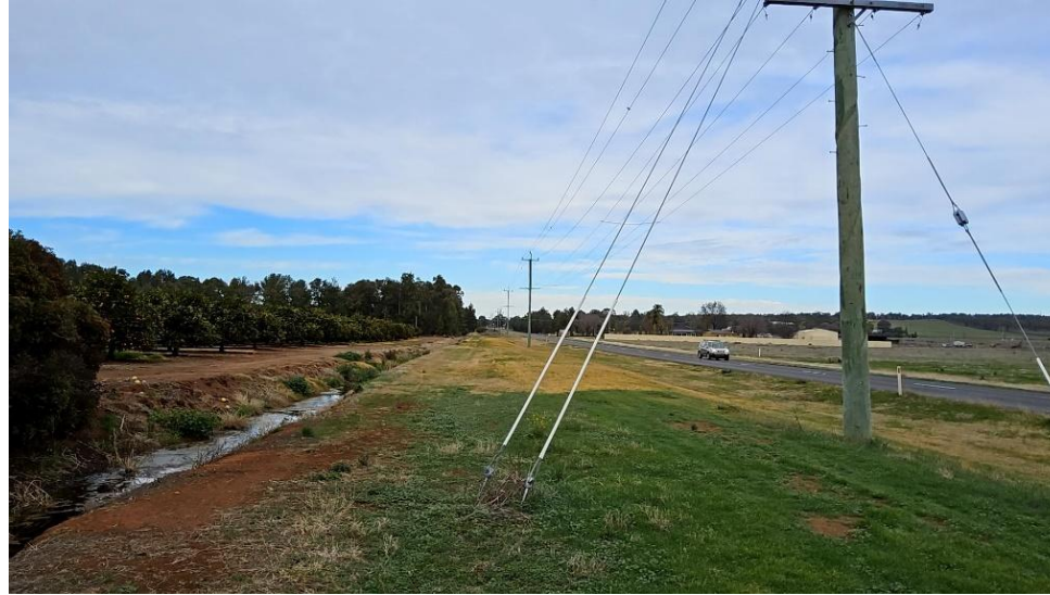
Figure 10: Extensive overhead infrastructure
