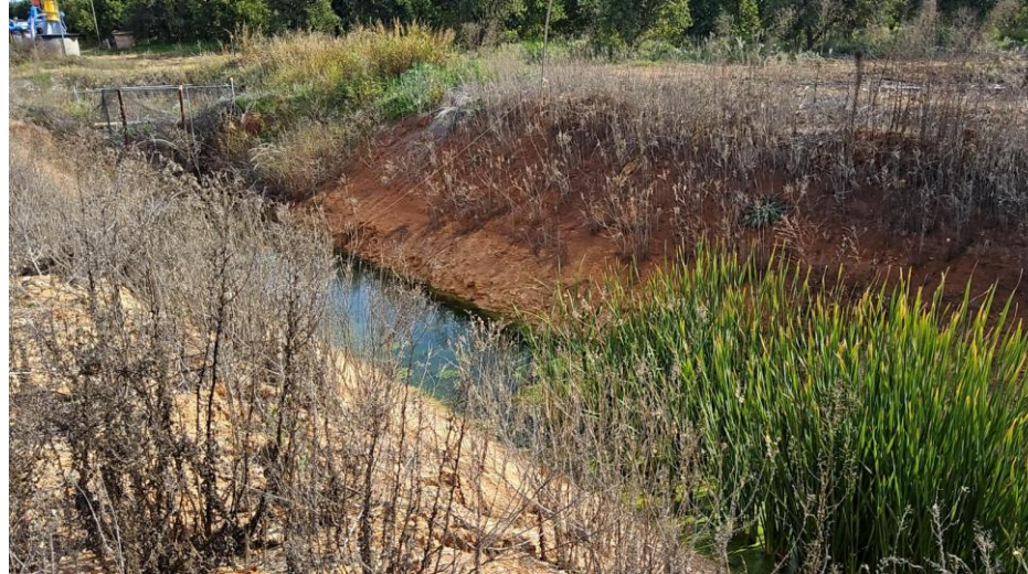
Figure 7: Existing channel near west end of Druitt St
